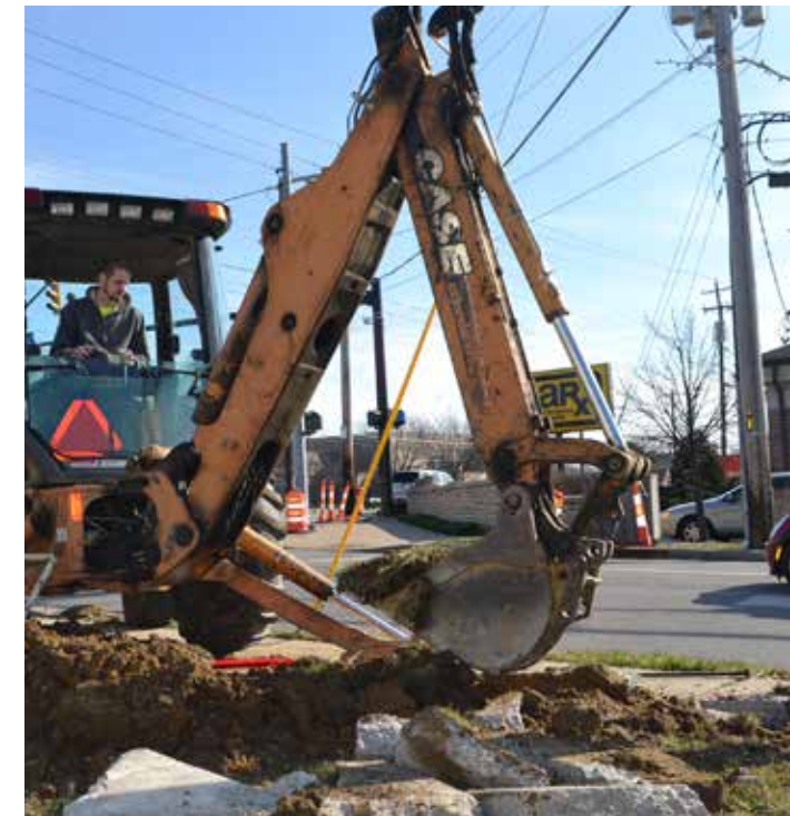
Sidewalk construction on Beechmont Avenue
